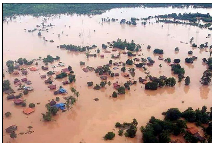
Figure 5.7: Downstream flooding following the collapse of Saddle Dam D in Lao PDR.
